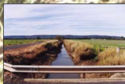
Typical drainage canal
